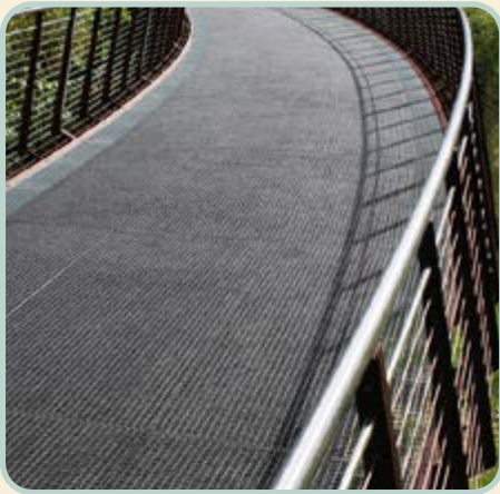
Fibre reinforced plastic (FRP) boardwalks
