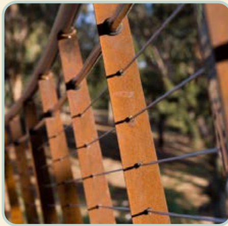
Balustrade in stainless steel and weathering steel
