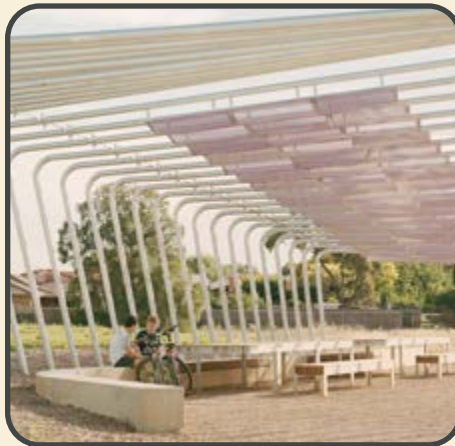
Concrete and steel for durability. Timber to provide tactility and comfort
